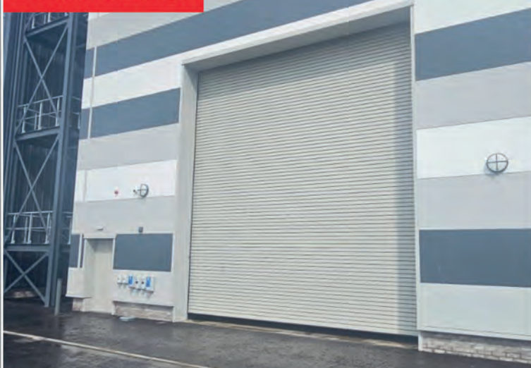
Vertically rolling industrial access door Rw30dB, Rw31dB, Rw53dB
