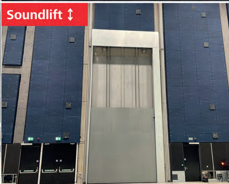
Vertical composite leaf sliding acoustic access door from Rw41dB to Rw58dB
